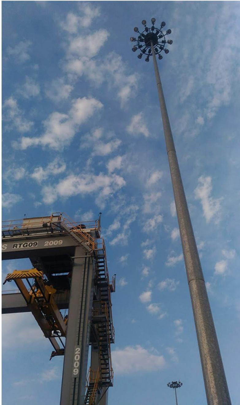
Figure 34: HMLP where Radios and Antennas can be Installed Only on the Metal ring at the Top of the pole
