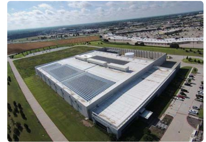
Cisco's Allen, Texas, Data Center Solar Project
